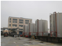
MMA storage tank
